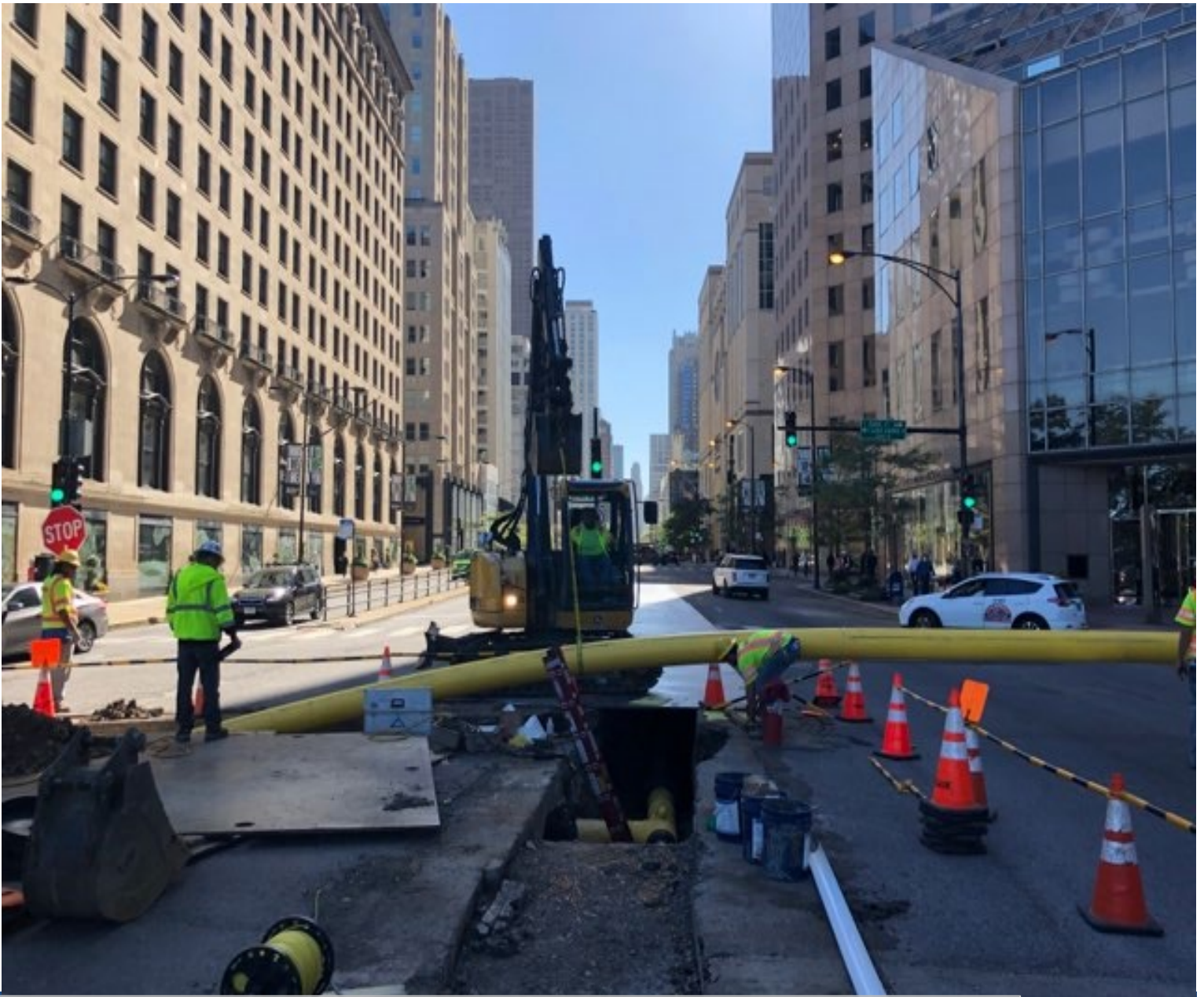
New main installation at Michigan and Oak.
